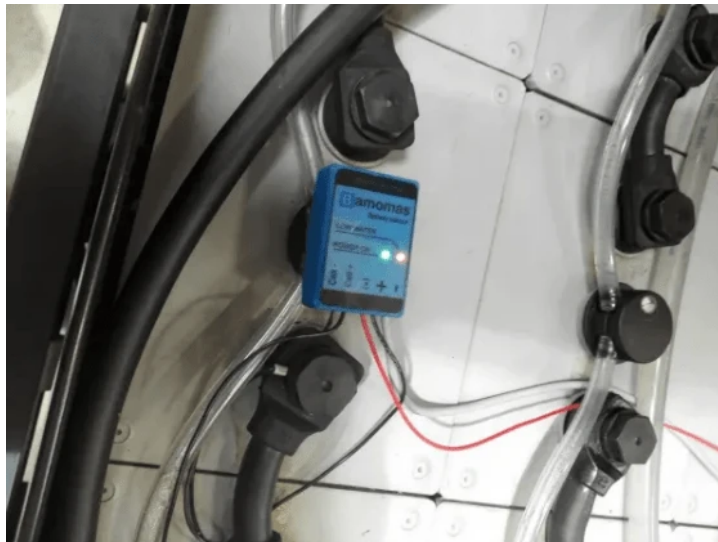
Figure 4.4.1: Bamomas lead-acid battery sensor device, Source: Bamomas Battery Intelligence Oy
